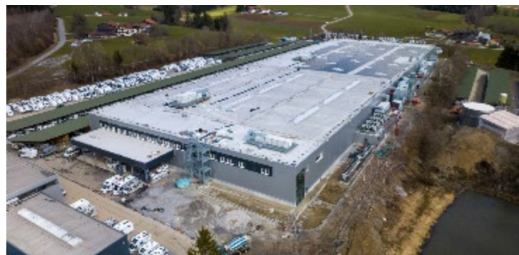
JANDELBRUNN (HQ) GERMANY
